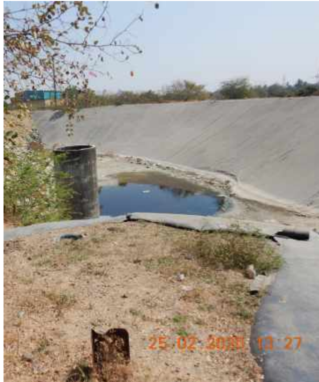
Plate 7.5.2: Photo showing active land fill pit and leachate monitoring well
