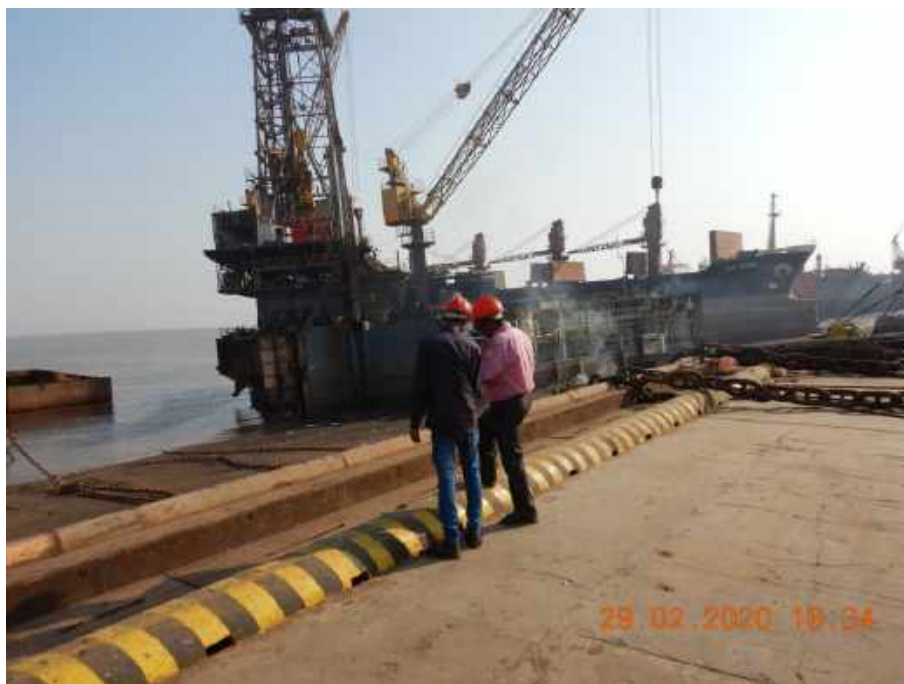
Plate 7.3.4: A view showing Green category yards with concrete flooring
