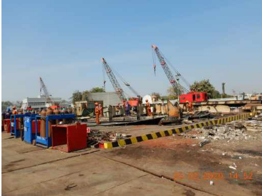
Plate 7.6.1: Workers working with almost all safety equipment
