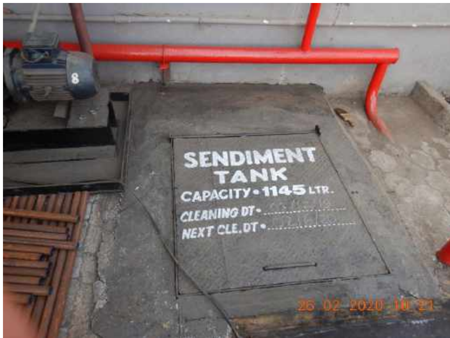
Plate 7.3.6: Photo showing sediment collection tanks constructed in yards to arrest sediment of the plot
