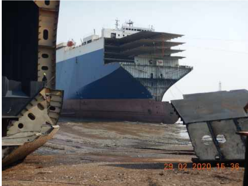
Plate 8.1.4: Photo showing ship cutting activities in the CRZ-I(B) region
